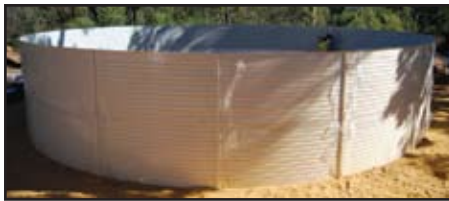
Completion of second ring
