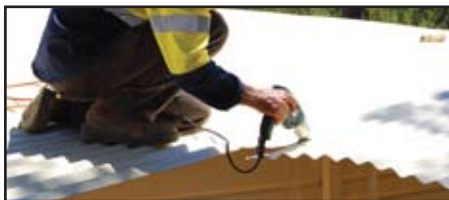
Trimming roof sheets to roof diameter
