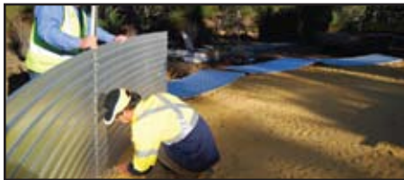
Construction of first ring
