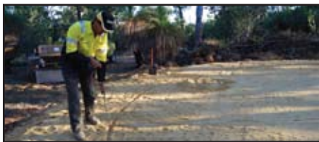
Marking out tank diameter
