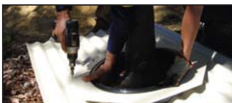
Fitting the filter basket
