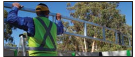
Fitting dome trusses
