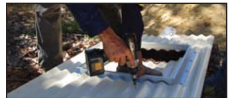
Fitting the access hatch
