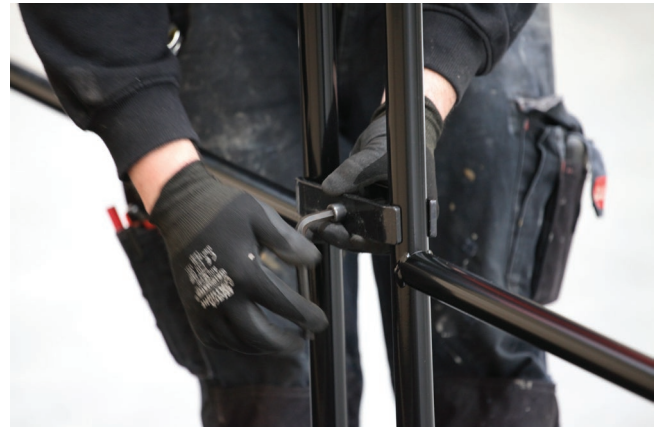
Once all Hand Rails are secured and joined add a Rail Clamp to each adjoining Hand Rail and Hand Tighten
