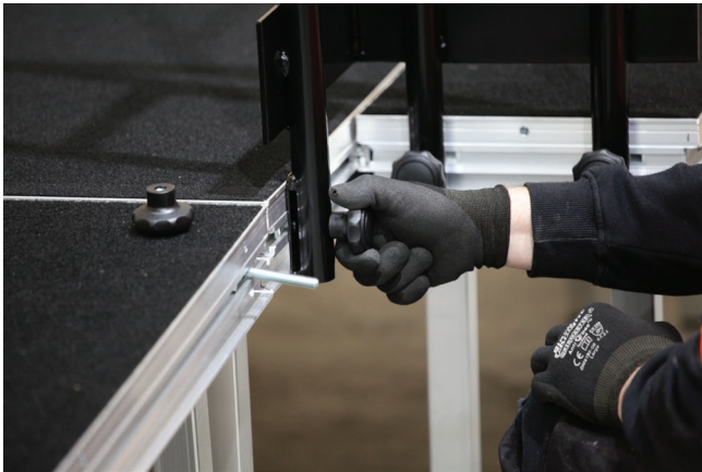
On Top Landing start with Corner Hand Rail
