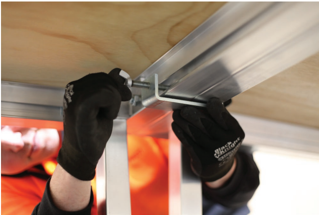
Attach the 2 Ramp Clamps under the Landing and Ramp Podiums - Clamp and Hand Tighten
