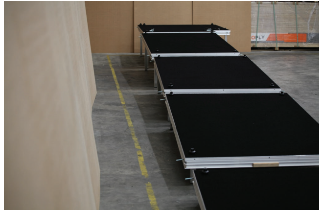
Add 2 T-Bolts per Ramp Podium ready for the Hand Rails
