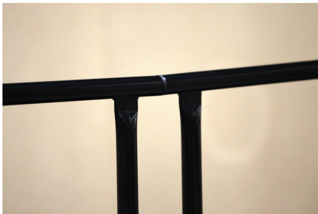
Slide a Hand Rail Joiner between 2 Hand Rails and push to secure
