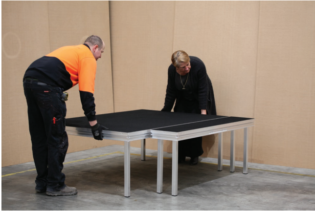
Position the 1.2m x 300mm Podium against the Stage then place the 1.8m Landing Podium next to the 1.2m Podium
