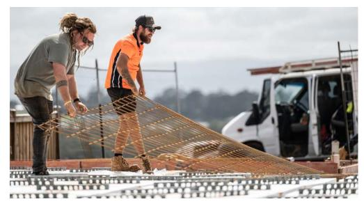
**PLACE PODS AND STEEL REINFORCEMENT** Install the waffle pods, pod rails/bar chairs, and steel mesh and bar.
