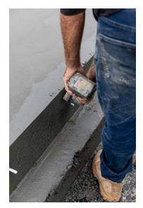
**CUT OFF BOLT** Using an angle grinder, cut the bolt flush with the slab.
