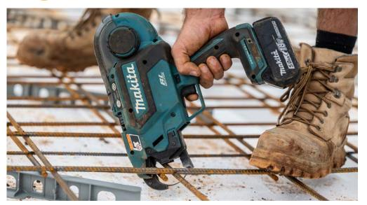
**TIE MESH** Tie the mesh in place with wire.
