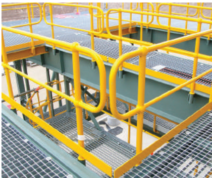
Balltube & Fabricated Handrailing
