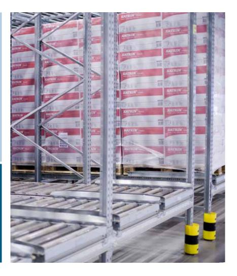
Pallet Flow Racking is a gravity fed storage system, which allows products to be loaded from the back and picked from the front. Once a carton is empty and removed from the rack the next box will roll to the front automatically. Also known as Pallet Live Storage, Pallet Flow Racking offers a First-In, First-Out (FIFO) storage flow, and uses 60% less space than standard, single entry pallet racking.
