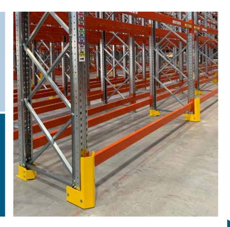
Twice as deep as selective racking, a Double Deep Pallet Racking configuration allows for the storage of two pallets per location and can be stored a maximum of 5 levels above the ground. This saves on aisle space and allows for an increased storage capacity in your warehouse.
