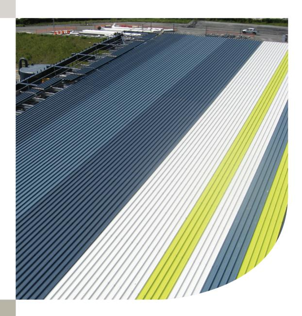
PERMALITE® products are made from marine grade aluminium, roll-formed to produce high performance cladding or purlins with an exceptional combination of strength and light weight.
